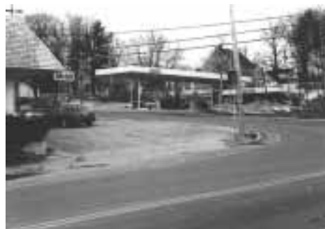
View of the Downtown Gateway from Bridge Street
